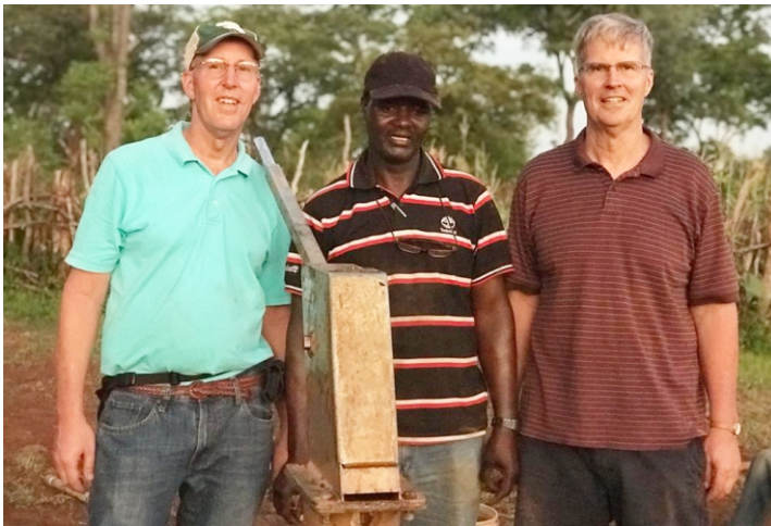
Brian with Cory and Simeon fixing a borehole in Livingstone
